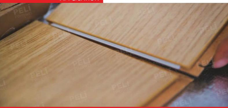
After the first panel is edged to the wall, the head lock system of the second panel is mounted at 45°.
