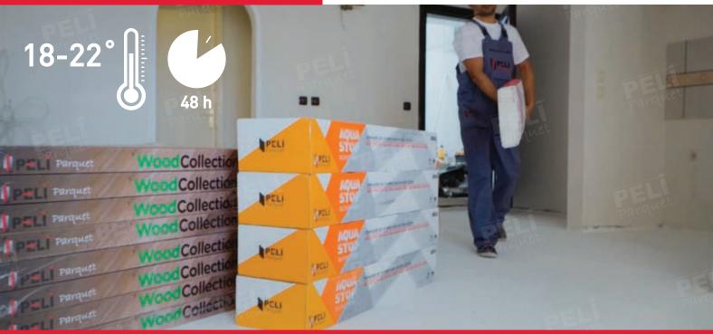
The products are transported to the parquet flooring area 48 hours in advance. The products are accustomed to the moisture in the environment. It is recommended to use aluminum foil underlay PELİ AQUA STOP, which has moisture barrier property, in new constructions or places where new screed application is applied. Problems caused by moisture that occur when not in use are not covered by the warranty.
