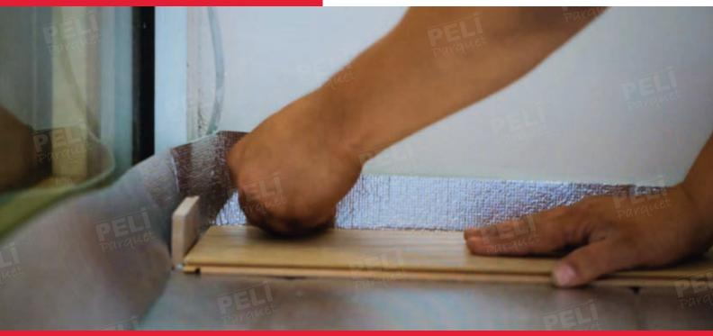
The PELİ ALJQA STOP aluminum foil underlay, which has a moisture barrier feature, should be folded up from the wall (6-8 cm) at the height of the baseboard to be used. This method of application also protects the baseboard against moisture coming from the wall.
