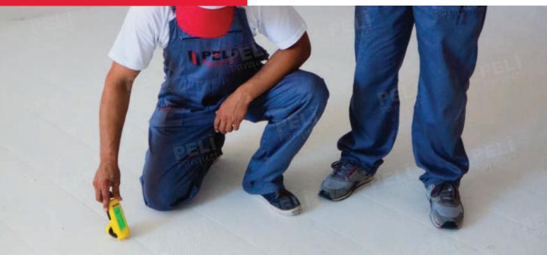
Floor moisture is checked. Humidity rate on the floor should not exceed 20%In cases with humidity rate above 20%, it is recommended to wait for the floor to dry and the humidity rate to decrease.
