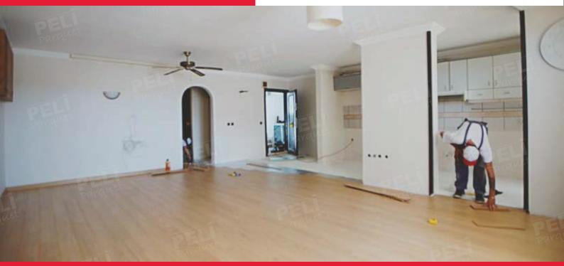
At the end of the application, transition profiles are attached to the joints when moving from the parquet to the other floor materials.
