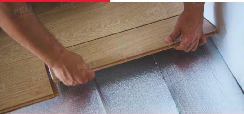
The difficulties encountered, especially when installing the last piece, are made much easier in parquets with UNIFIT lock system (head-end sealed locking system). The head lock system of the panel, which is attached at an angle of 45 °C from the side, is pressed from the top until the "click" sound is heard after being edged to the second panel.
