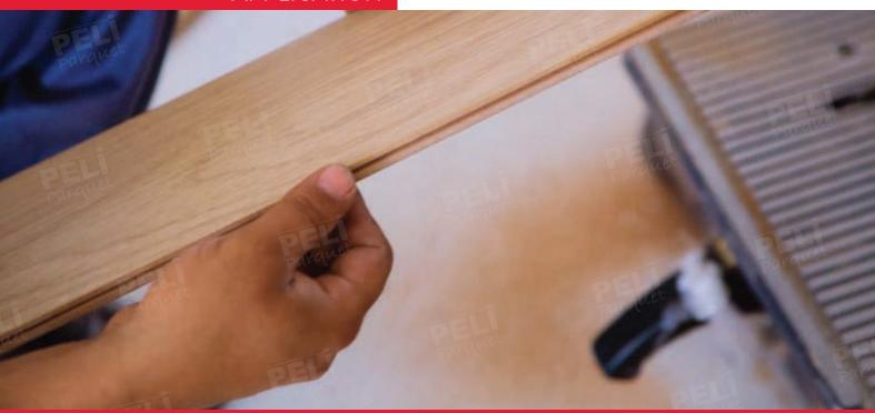
When starting the first row, the male lock side of the panel is machined off with the machine.
