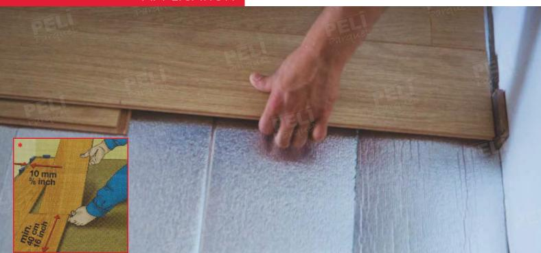
While attaching the last piece of each row, a gap is always left at an equal distance from the wall.
