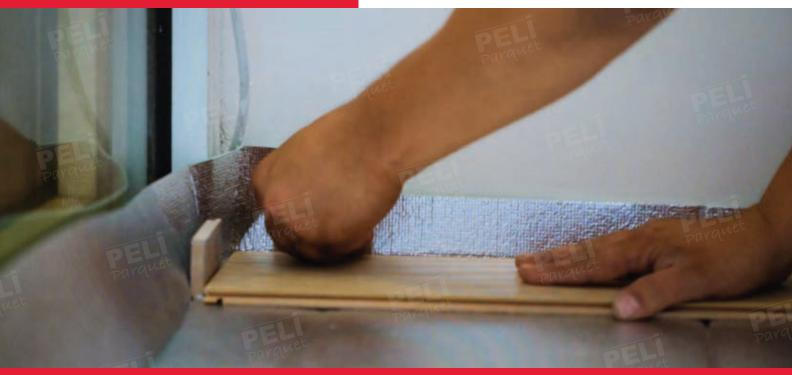
The panel in the first row is moved away from the wall both at the head and the side by using min. 16 mm wedges.
