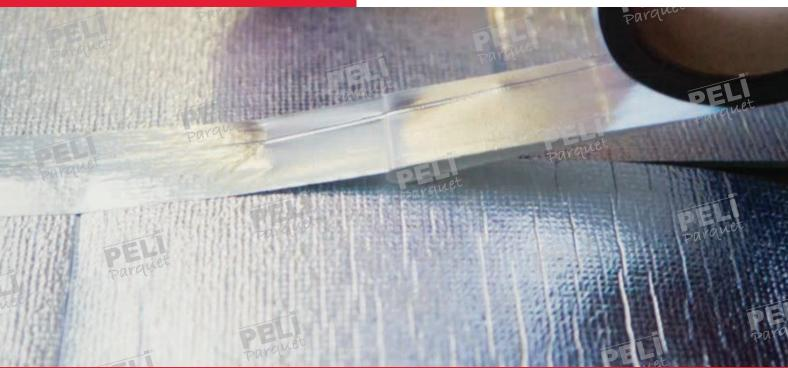
A underlay is laid on the floor first. A high level barrier against moisture that may come from the floor is created by tapping the joints with the 5 cm wide aluminum foiled tape included in the PELI AQUA STOP underlay box.
