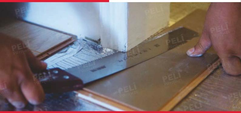
The lower part of the door-frame jambs is cut off with a hand saw to get a better appearance.
