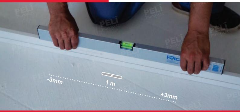
Floor control is made with a 2 meter gauge and water balance. Deviation at a distance of 1 meter should not exceed ± 3 mm.
